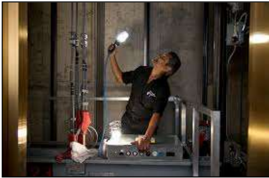
ELEVATOR SHAFT HOIST WAY CONDITION INSPECTION
