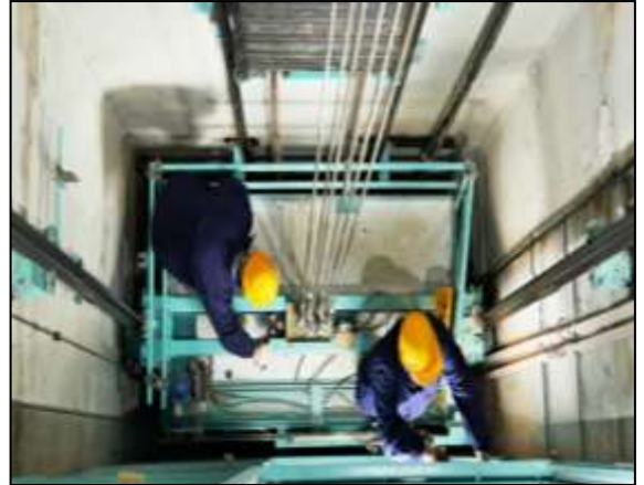
ELEVATOR CAR TOP CONDITION INSPECTION
