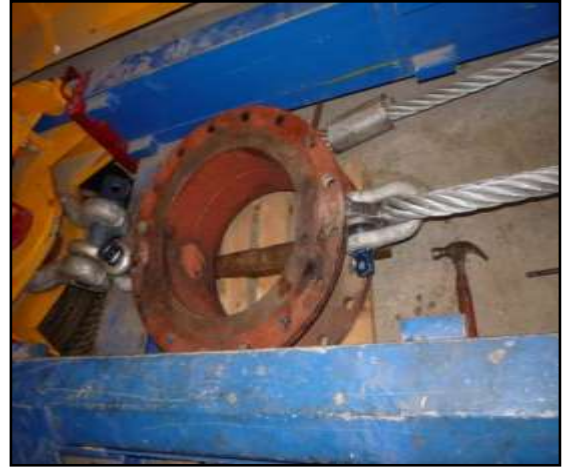
LOAD TEST OF LIFTING SPOOL PAD EYES @ 40 MT USING 75 MT TEST BENCH.
