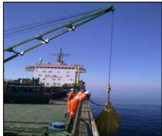
LOAD TEST OF DECK CRANE ONBOARD VESSEL "M.V.CORAL"
