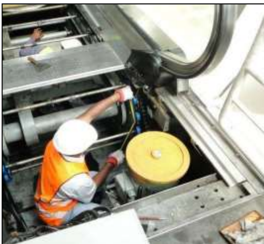
ESCALATOR & WALKS MACHINE FUNCTIONAL TESTING
