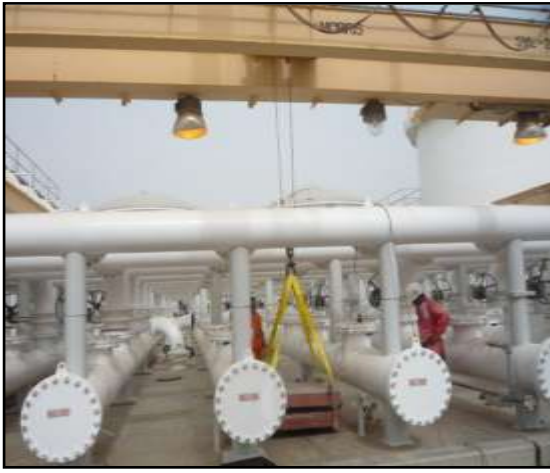
LOAD TEST OF OVERHEAD CRANE - USING CALIBRATED TEST WEIGHTS & LOAD CELL.
