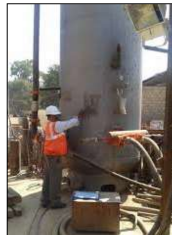
AIR RECEIVER VISUAL AND FUNTIONAL TESTING
